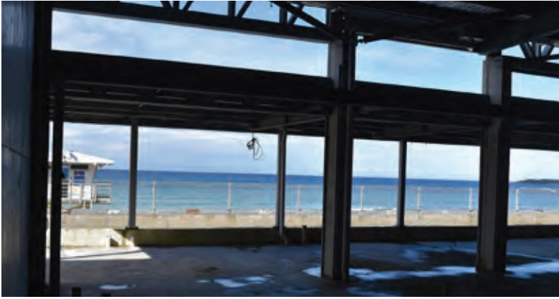
Level 1 and Patrol Tower
